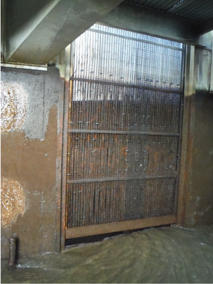
Photo 1. Adult trap recovery pool looking towards the sample basket and screen that plugged with shad mortalities during dewatering for shad July 10, 2017.
